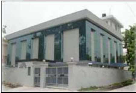
JPNATC/SMT Call Centre Building at NOIDA
